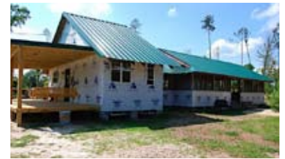
The dining hall undergoes repairs.
